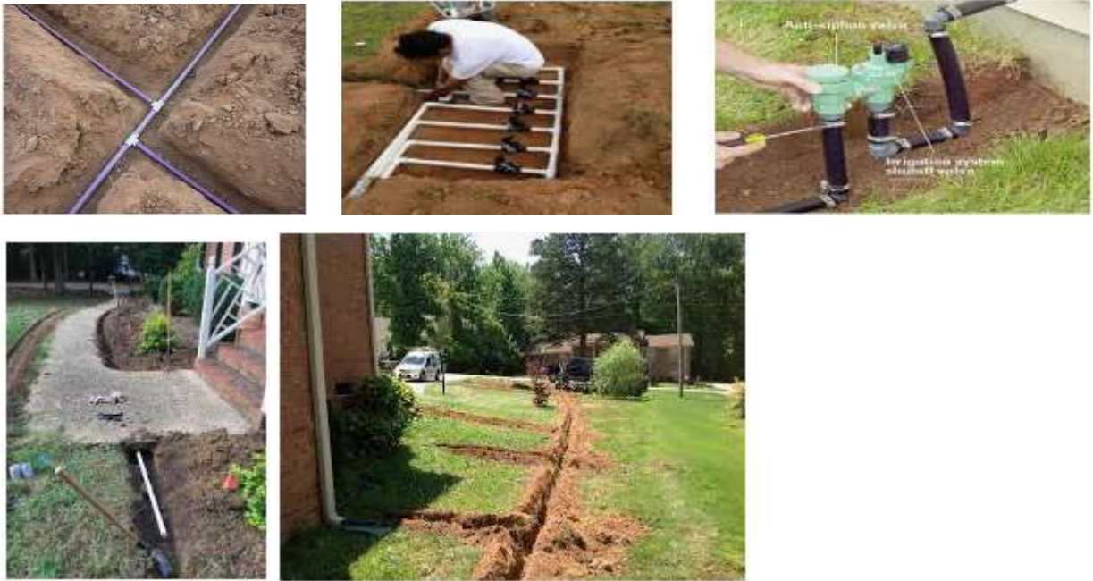
Fig.4 Different Images of pipe installation (Source: https://www.shutterstock.com > search > irrigation pipe )
